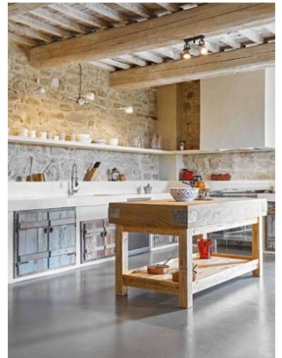
Rivestimento a pavimento con due mani di malta ecologica texture fine, spatolato e velato. Residenza privata, Italia / Floor covering with two coats of fine texture ecological mortar, brushed and veiled. Private residence, Italy.
